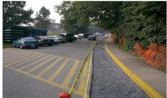
(from left to right) Installation of Inlets and Control Structure; Non-woven Geotextile is folded over Infiltration Trench; Stabilized Site
