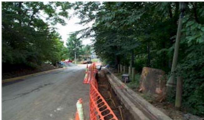
(from left to right) Installation of Inlets and Control Structure; Non-woven Geotextile is folded over Infiltration Trench; Stabilized Site
