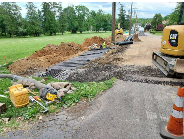
Ready for the trench to be backfilled.
