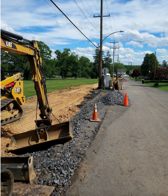
Earth is replaced.
