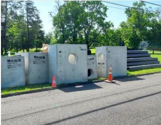
Construction supplies delivered on-site.
