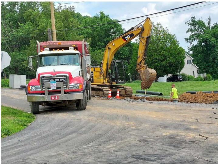
Digging the trenches.
