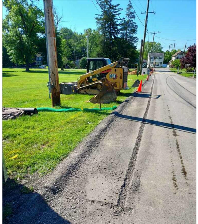
The old asphalt curbing was cut away and removed.
