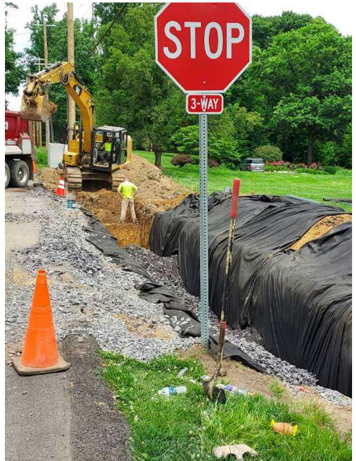
Infrastructure being installed.
