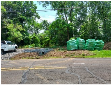
Pipes are placed to redirect stormwater from Hill Ave.
