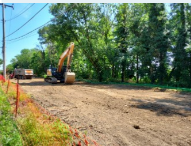
Ground is leveled and ready for excavation.
