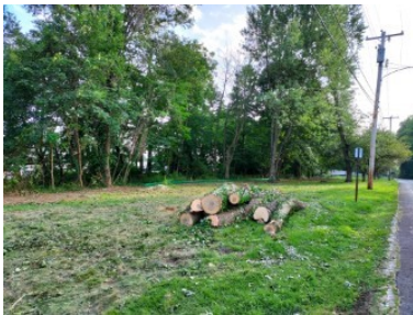
Trees are cleared to make way for the basin.
