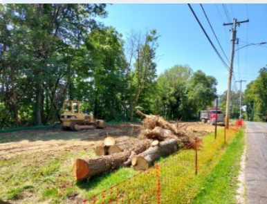
The ground is beginning to be leveled
