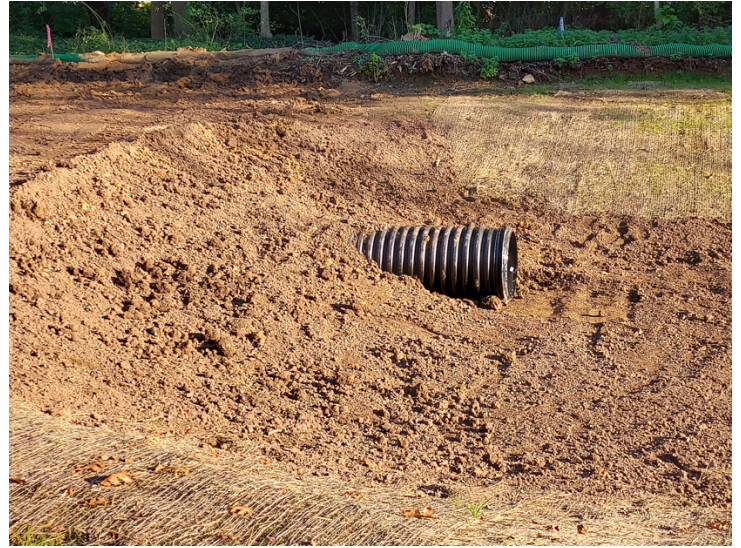
Pipe is placed connecting the two basins
