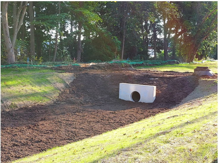
Headwall is placed at exit of first basin
