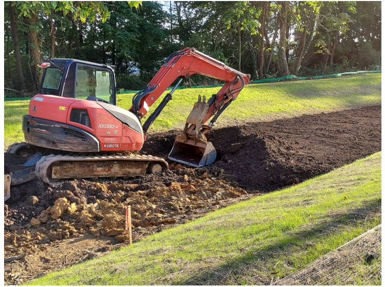
Amended soils are starting to be placed
