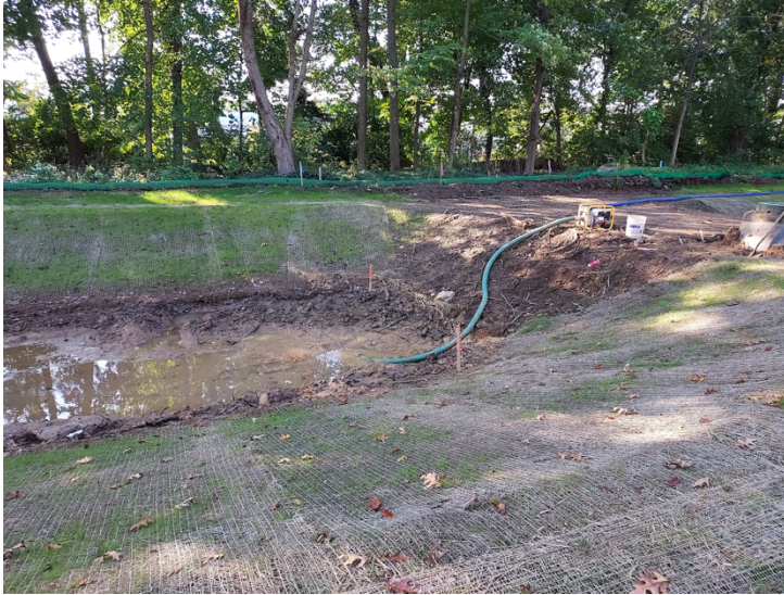
Water from recent rains is pumped out of the basin.
