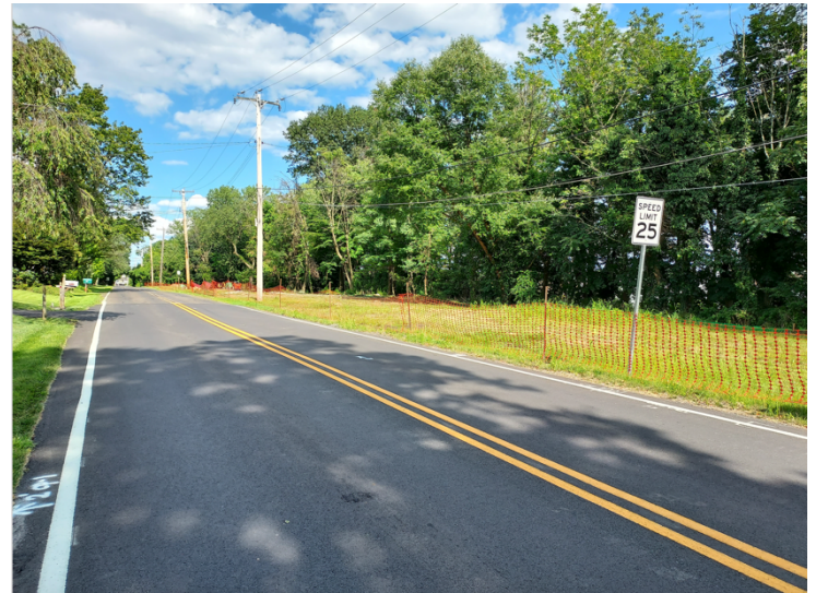
Construction fencing is placed around the site.
