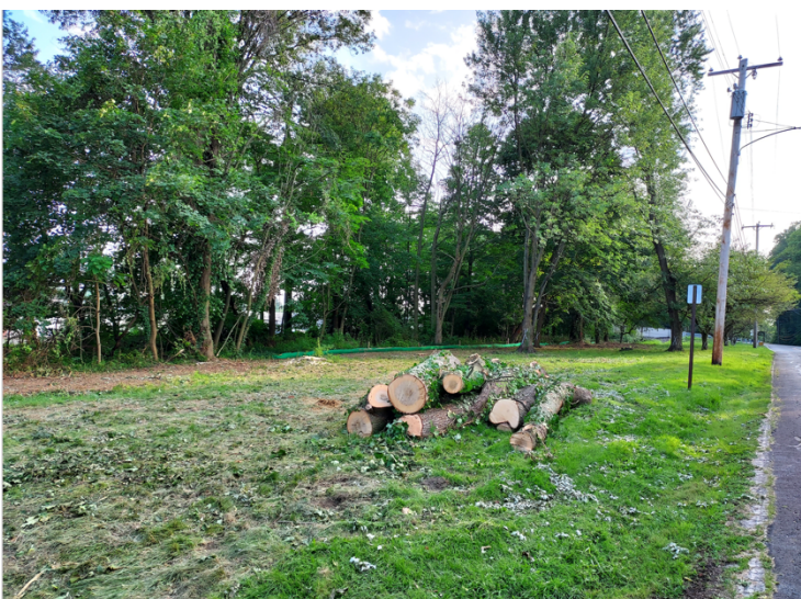
Trees are cleared to make way for the basin.
