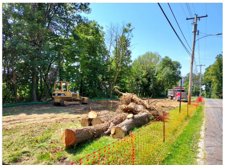
The ground is beginning to be leveled.
