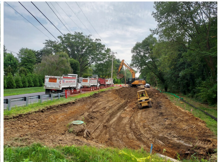
Excavation has begun.
