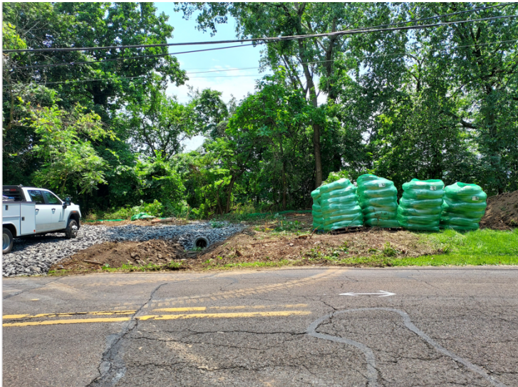
Pipes are placed to redirect stormwater from Hill Ave.
