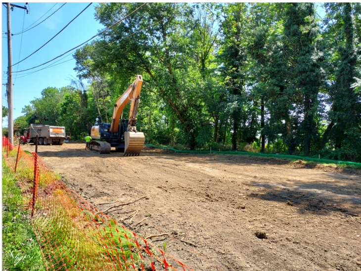
Ground is leveled and ready for excavation.
