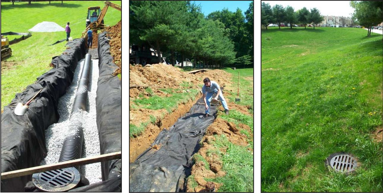
Figure 6.4-6. (From left to right) Installation of Inlets and Control Structure; Non-woven Geotextile is folded over Infiltration Trench; Stabilized Site
