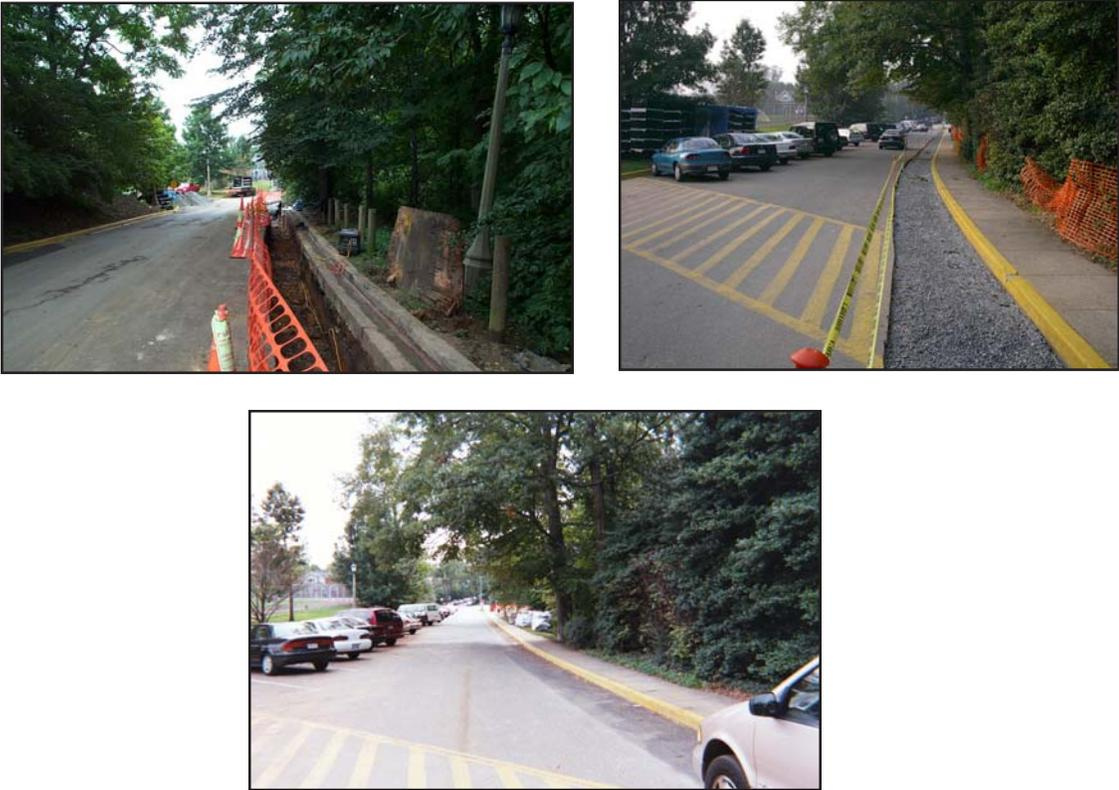
Figure 6.4-7. (Clockwise from top left) Infiltration Trench is on downhill side of roadway; Infiltration Trench is Installed; Infiltration Trench is paved with standard pavement material
