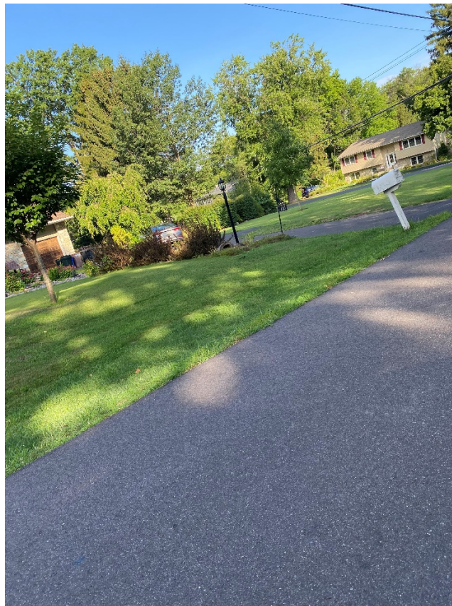
Picture 8: Hill Avenue Swale, in between Highland Avenue and Prospect Avenue
