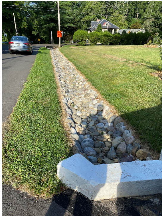
Picture 6: West Prospect Avenue Swale, in between Station Avenue and Hulmeville Avenue
