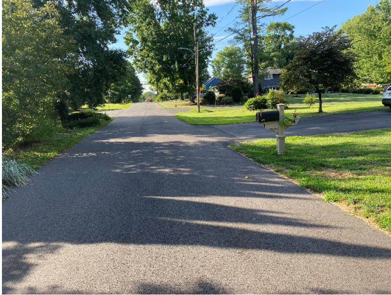
Picture 7: Hill Avenue Swale, in between Highland Avenue and Prospect Avenue
