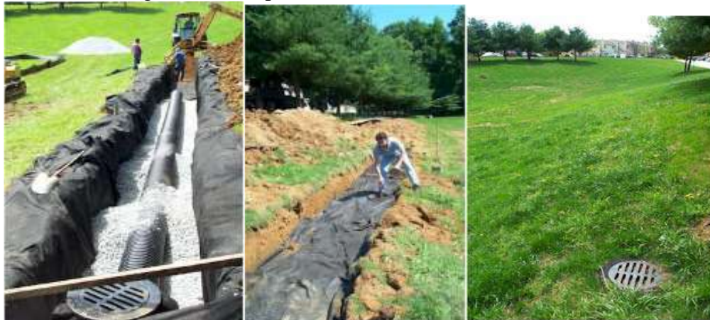
Figure 4: Example of Infiltration Trench Installation
