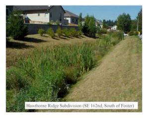
A Vegetated Swale is a broad, shallow, trapezoidal or parabolic channel, densely planted with a variety of trees, shrubs, and/or grasses. It is designed to attenuate and in some cases infiltrate runoff volume from adjacent impervious surfaces, allowing some pollutants to settle out in the process. In steeper slope situations, check dams may be used to further enhance attenuation and infiltration opportunities.
