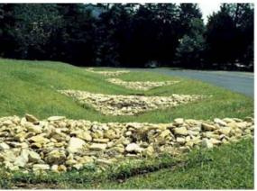
check-dam, a better approach might be to allow low flows (2-year storm) to drain through the stone, while allowing higher flows (10-year storm) drain through a weir in the center of the dam. Flows through a stone check-dam are a function of stone size, flow depth, flow width, and flow path length through the dam. The following equation can be used to estimate the flow through a stone check dam up to 6 feet long:
